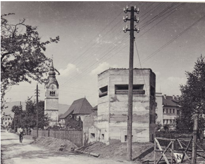
Bunker in Lesce (Lees)
